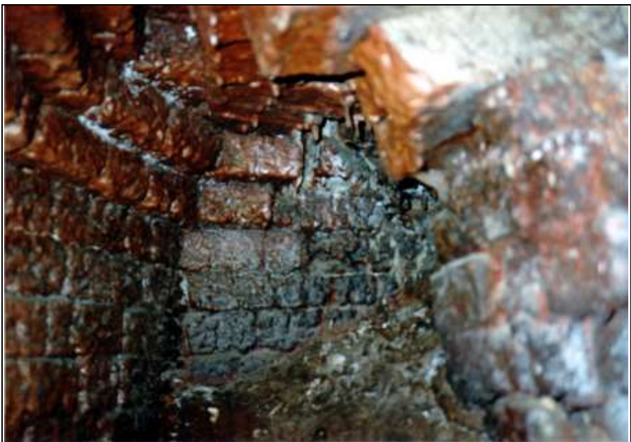
Photograph 5: Left-hand gasifier: Inside view, with the first opening connecting it to the left-hand muffle. The refractory brickwork shows evidence of fusion. (For two similar images, see Photographs 315f., which were placed later out of order.)
