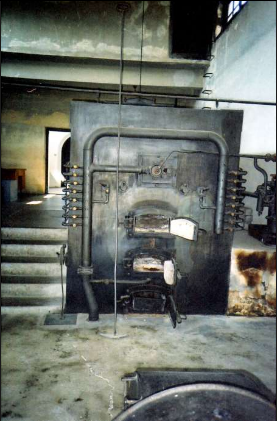
Photograph 348: as above, rear view.
