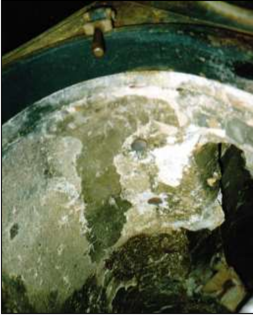
Photograph 41: Vaulted ceiling of the left-hand muffle; to the right: outlets of pipes connected to the blower.
