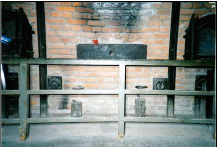
Photograph 289: as above; first recuperator.
