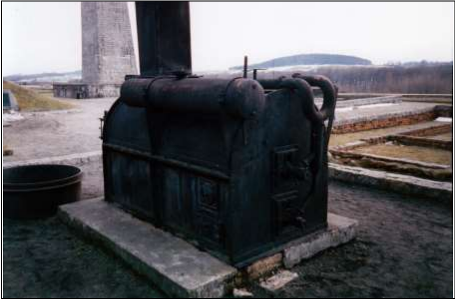
Photograph 333a: rear view. Top left: naphtha tank; below it: combustion-air inlet and access door; top right: combustion-air pipes; rear end: main (top) and auxiliary burner (bottom).
