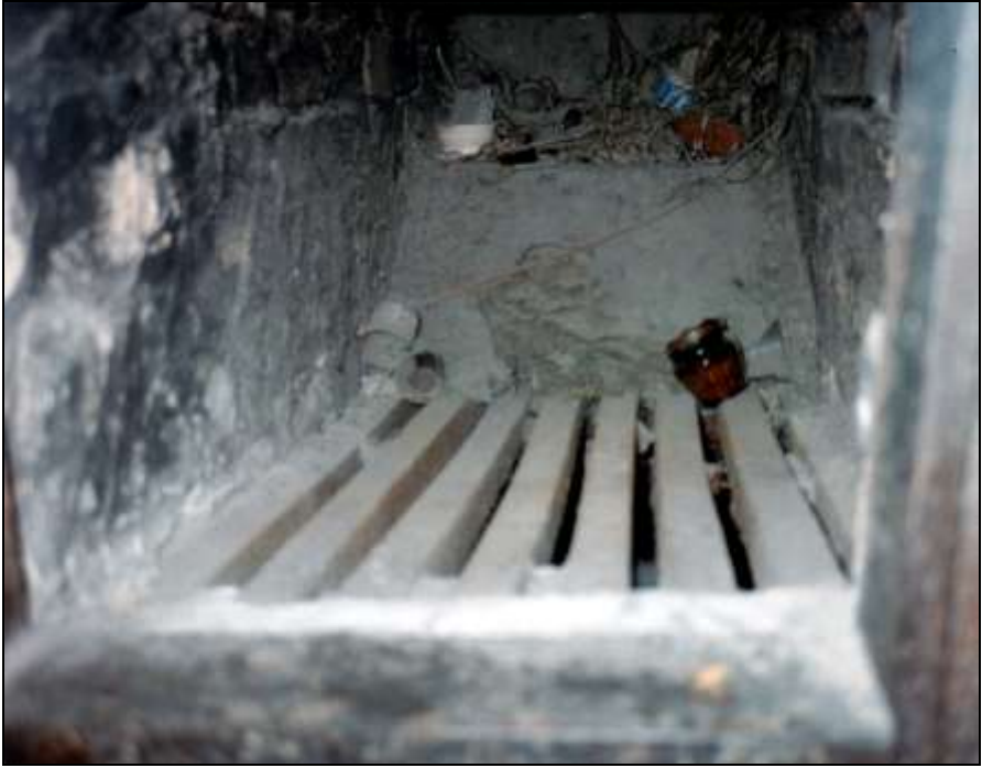
Photograph 99: Furnace No. 2: original gasifier grate with seven longitudinal bars and two transverse bars.
