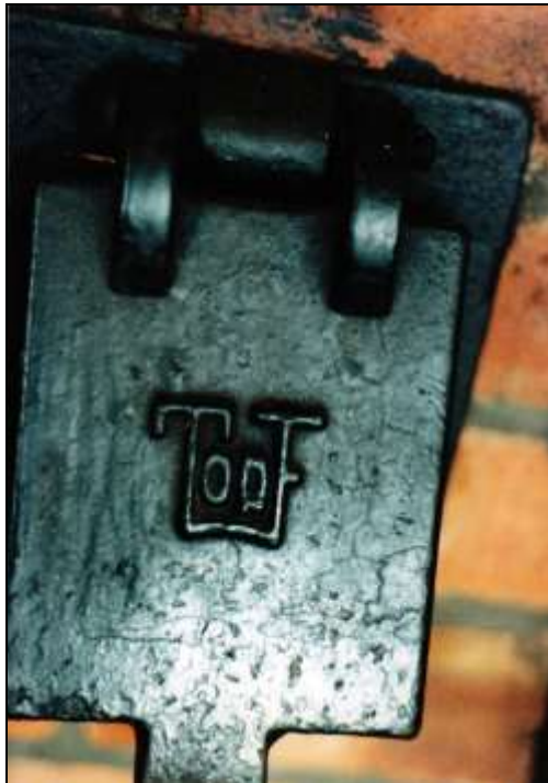
Photograph 154: combustion-air-channel door with the Topf logo, close-up.
