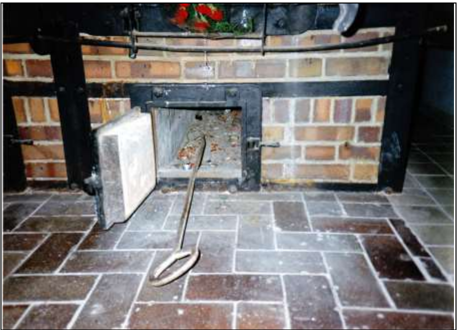
Photograph 71: Ash chamber of the right-hand muffle.
