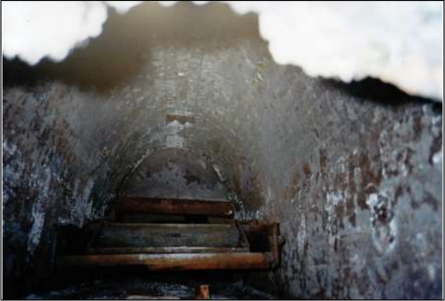
Photograph 352: as above; the muffle's interior seen from its rear service door. In the foreground the front part of the corpse-introduction cart.
