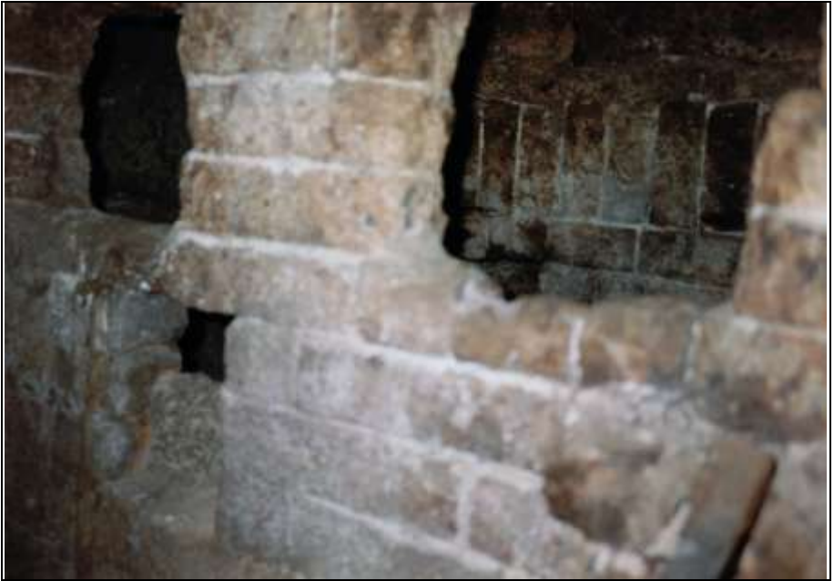
Photograph 20: Left-hand muffle: partition wall with inter-muffle openings.
