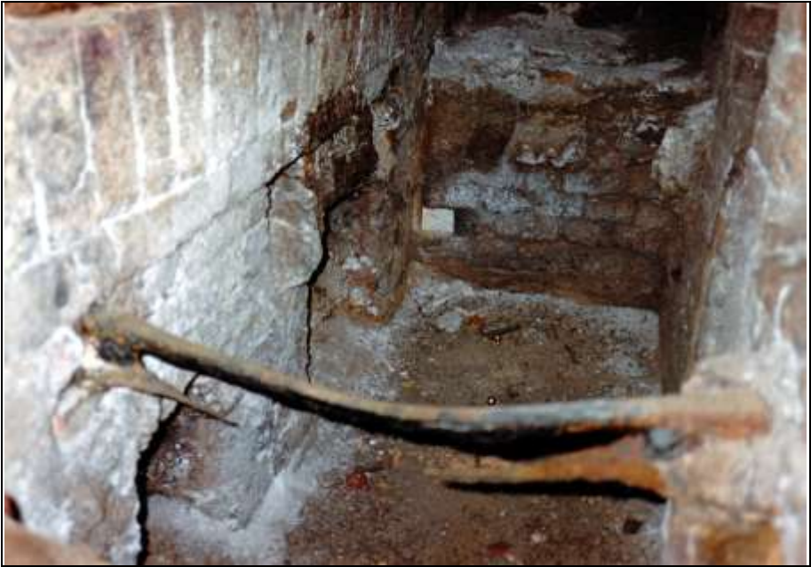
Photograph 16: Left-hand muffle: ash compartment with two openings connecting it to the gasifier.
