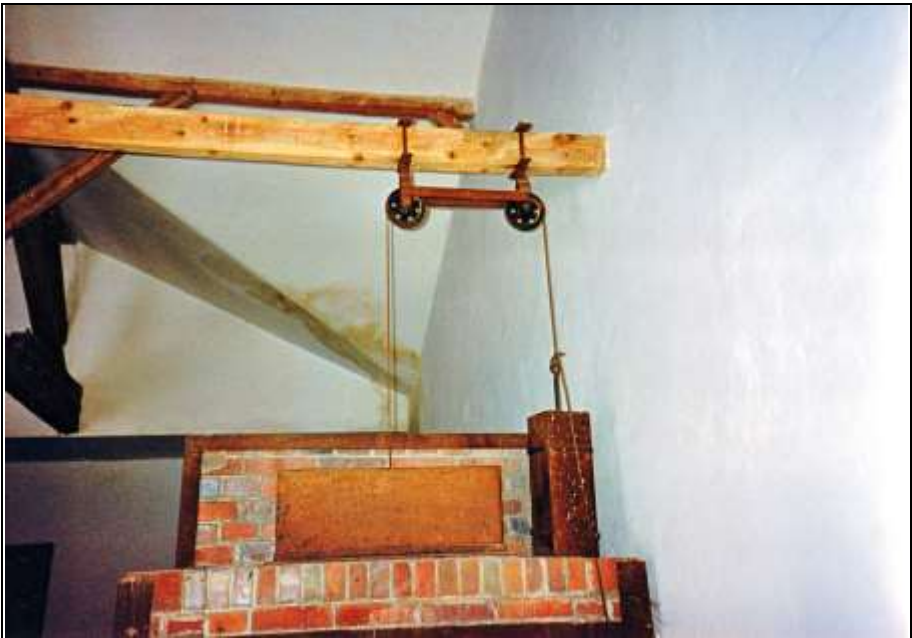
Photograph 255: Fourth furnace, front view: metal housing of the muffle door's corpse-retaining plate made of refractory clay; wire cable, pulley and counterweight for its operation.
