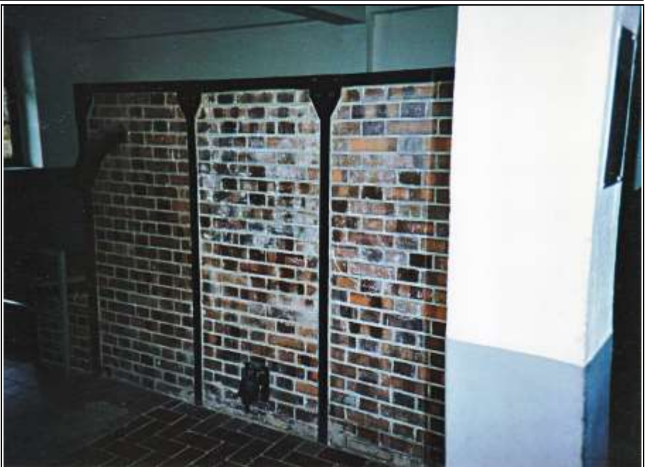
Photograph 73: Left side of the furnace: Door of the combustion-air-intake channel whose channel leads into the ash chamber of the left-hand muffle.
