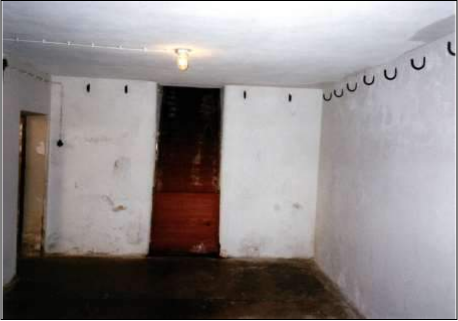
Photograph 210: as above; basement morgue, wooden corpse chute.
