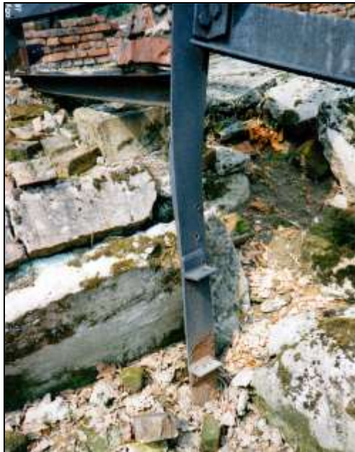
Photograph 231: as above. Detail of the north gasifier's frame irons (direction south-north). The two brackets visible below were used for mounting the gasifier's hearth door.
