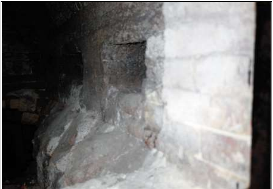
Photograph 134: as above, right-hand muffle wall with rectangular openings connecting this side muffle to the center muffle.
