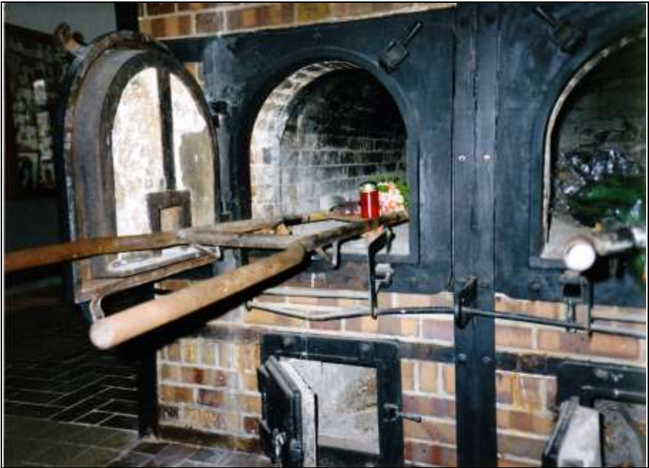
Photograph 69: Left-hand muffle with open ash door.
