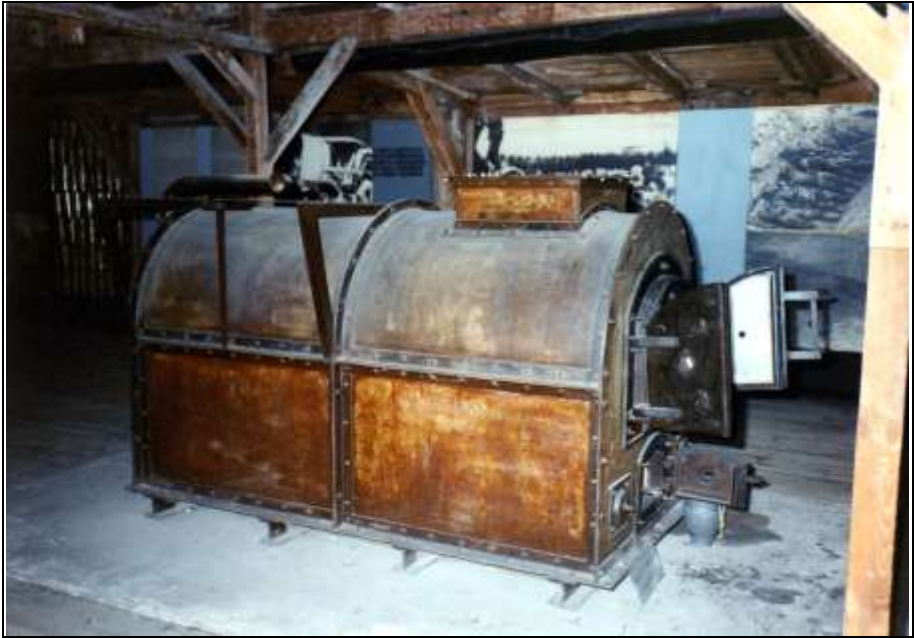
Photograph 324: left-hand side of the furnace.
