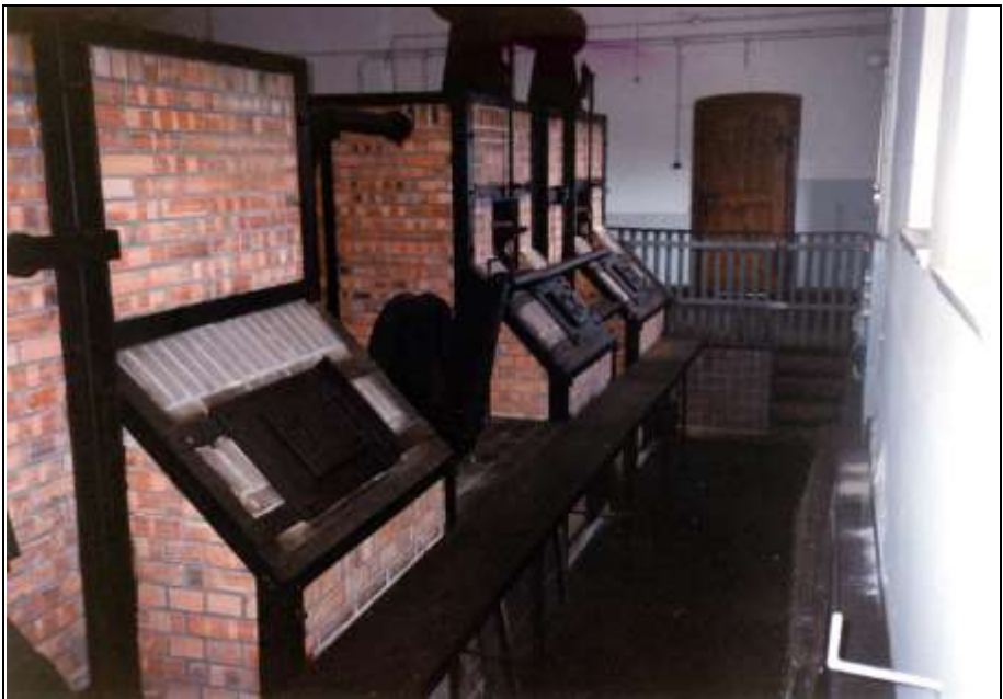
Photograph 158: TOPF triple-muffle cremation furnaces; right-hand rear view with the gasifier's coke-loading doors (top) and ash doors in the service pit (bottom).
