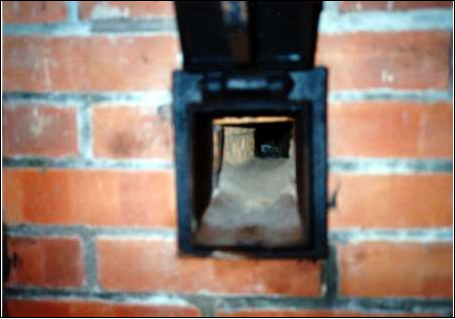
Photograph 171: as above; close-up of the ash chamber's combustion-air channel
