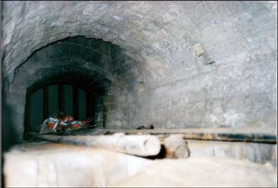
Photograph 279: Inside of the muffle seen through the main gasifier's coke-loading door. In the right-hand wall: openings for combustion-air supply. Top in the background: the opening of the smoke-gas outlet.
