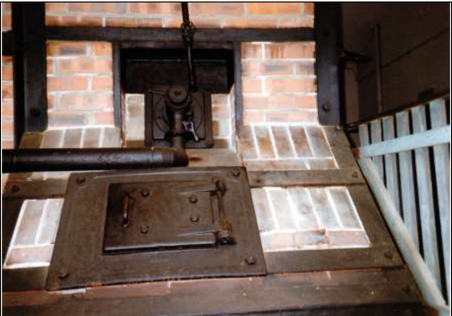
Photograph 160: TOPF coke- or naphtha-fired triple-muffle cremation furnace. Rear view, left-hand muffle. Naphtha burner (top) and the gasifier's coke-loading door (bottom).
