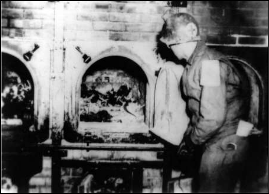
Photograph 206: A U.S. soldier in front of the central muffle of the TOPF coke- or naphtha-fired triple-muffle cremation furnace at Buchenwald Camp. U.S. Army photo of 1945.
