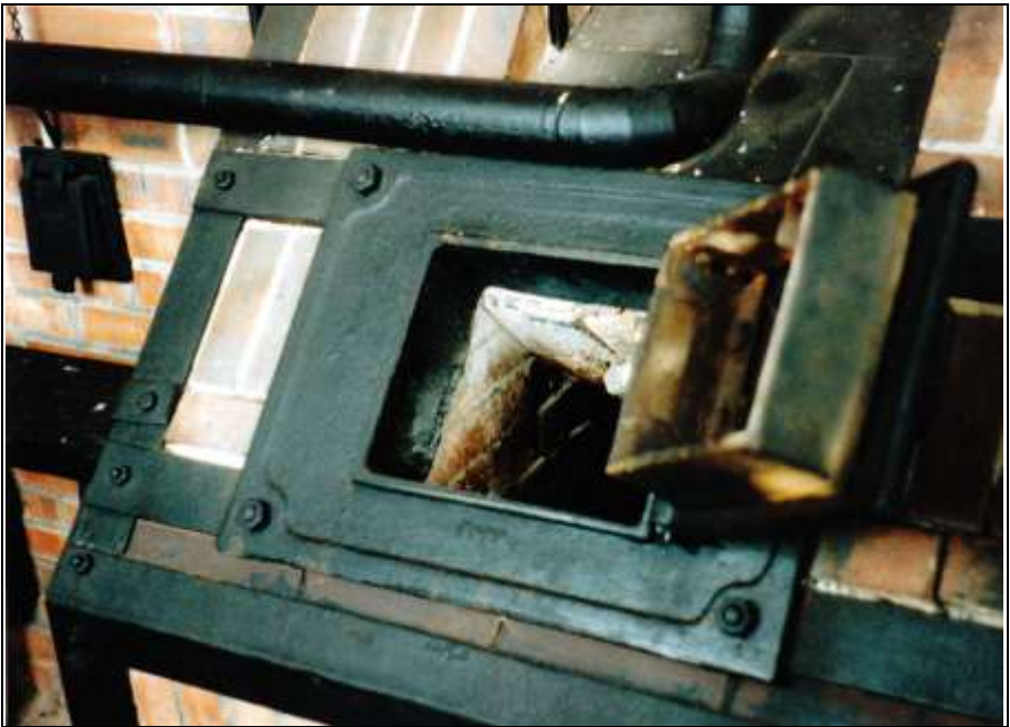
Photograph 162: as above, with opened coke-loading door.
