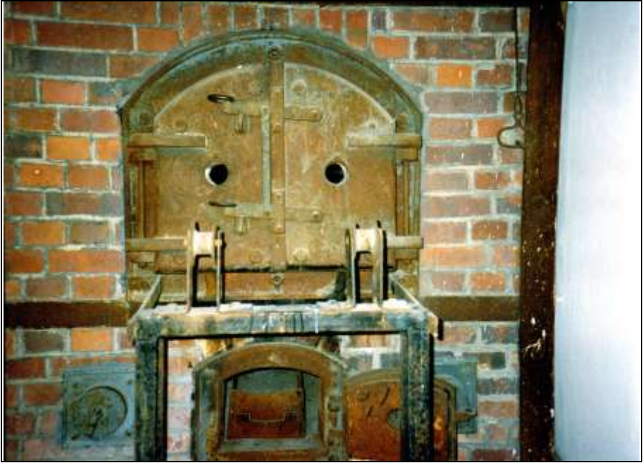
Photograph 250: The fourth furnace, muffle door.
