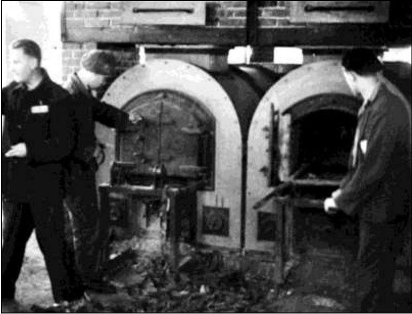
Photograph 342: KORI naphtha-fired cremation furnaces at Neuengamme Concentration Camp. Source: www.kz-gedenkstaette-neuengamme.de/typo3temp/pics/5f467c62d5.jpg , now removed
