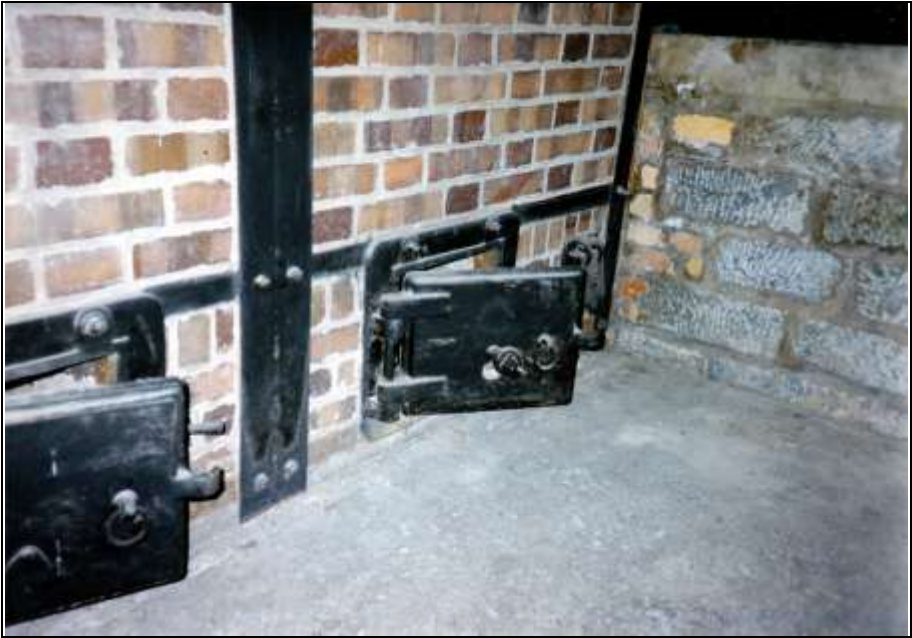
Photograph 80: as above, the gasifiers' ash-chamber doors.
