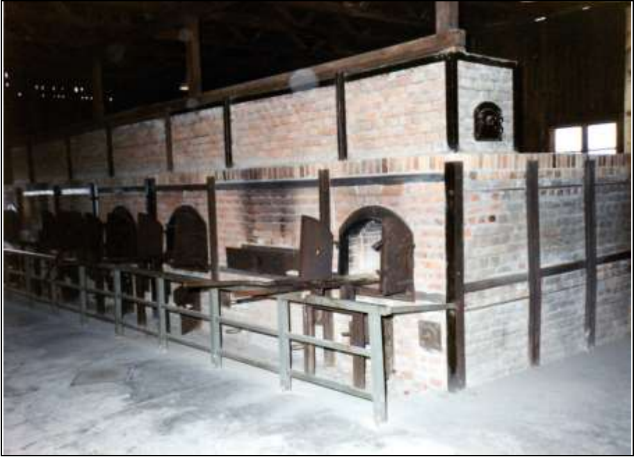
Photograph 309: Front view from the right-hand side. The brick structure at top contains the smoke duct, with an inspection door on the side.
