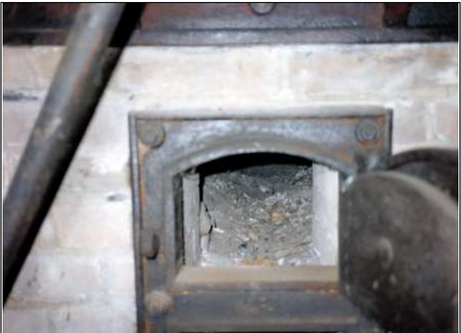
Photograph 303: Access door to the post-combustion area.
