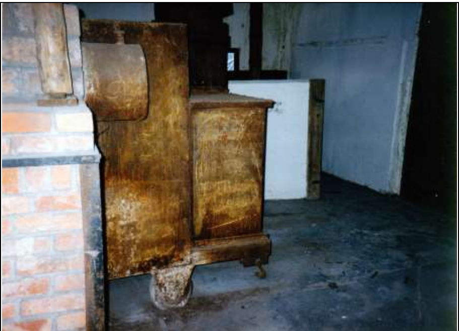
Photograph 46: Rear side of the furnace seen from the right: Fuel tank (top left) and metal wheels of the furnace body (bottom).
