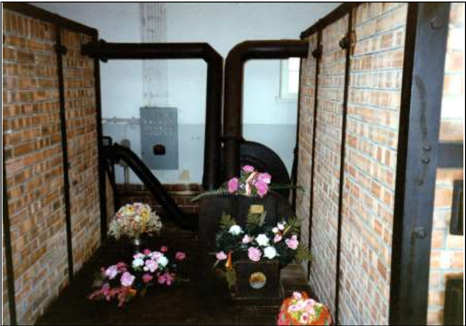
Photograph 188: Blowers located between the two furnaces.
