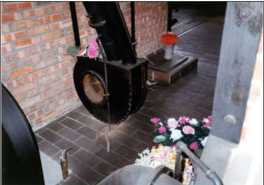
Photograph 190: as above, rear view.
