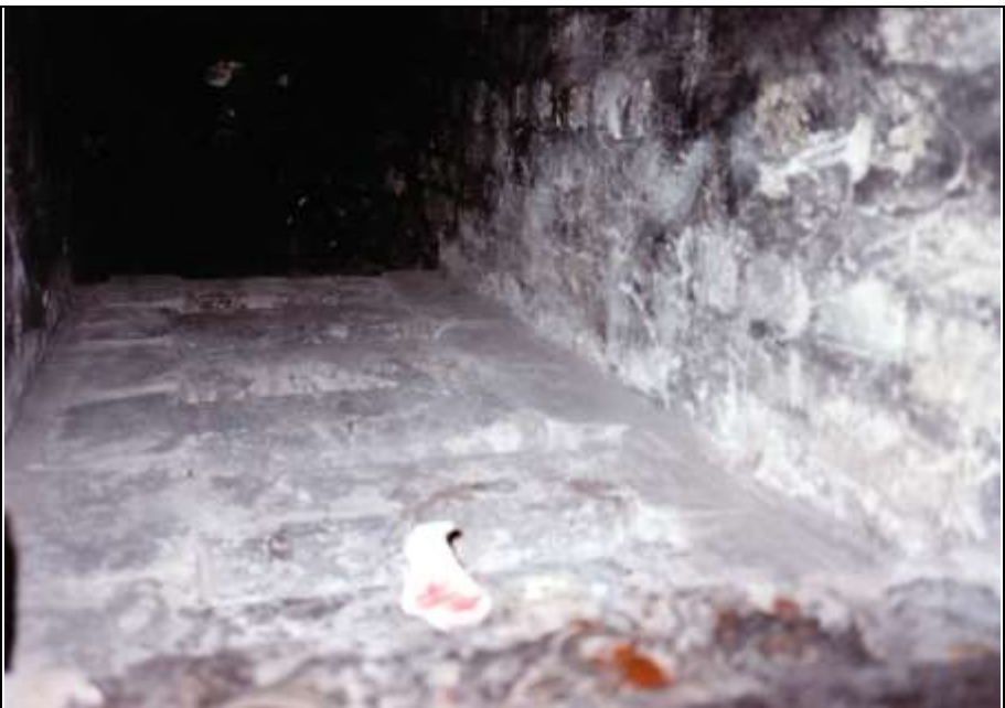
Photograph 93: Furnace No. 2: grate of the left-hand muffle.
