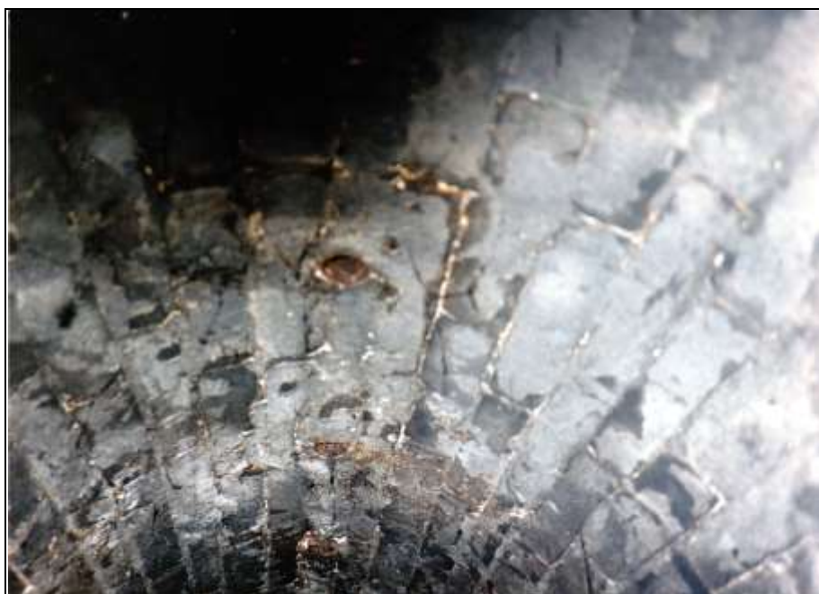
Photograph 61: Vaulted ceiling of the right-hand muffle; outlets of pipes connected to the blower.
