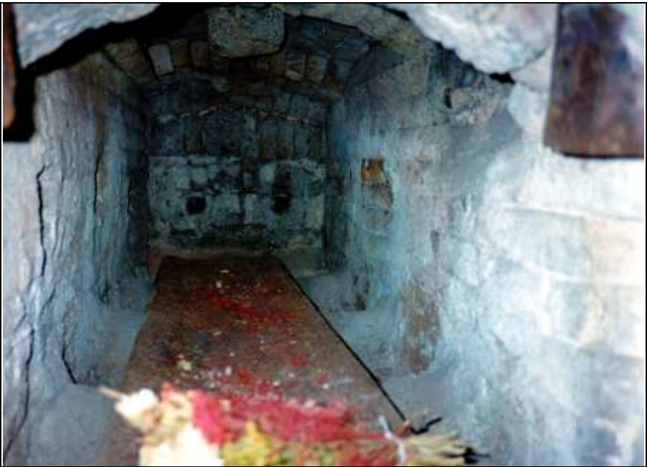
Photograph 239: Inside the muffle.
