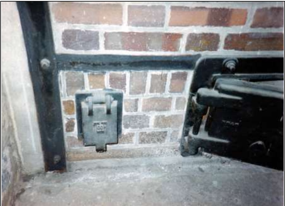
Photograph 81: as above; the left-hand combustion-air-intake door.
