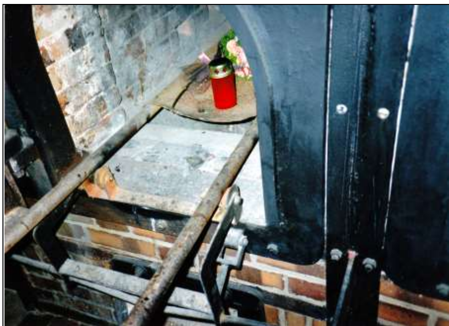
Photograph 85: as above, viewed from top: the movable roller device on which the bars of the corpse stretcher rests.
