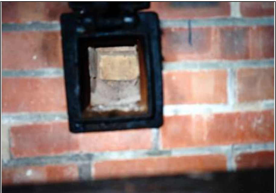
Photograph 170: as above; close-up of the muffle's combustion-air channel.
