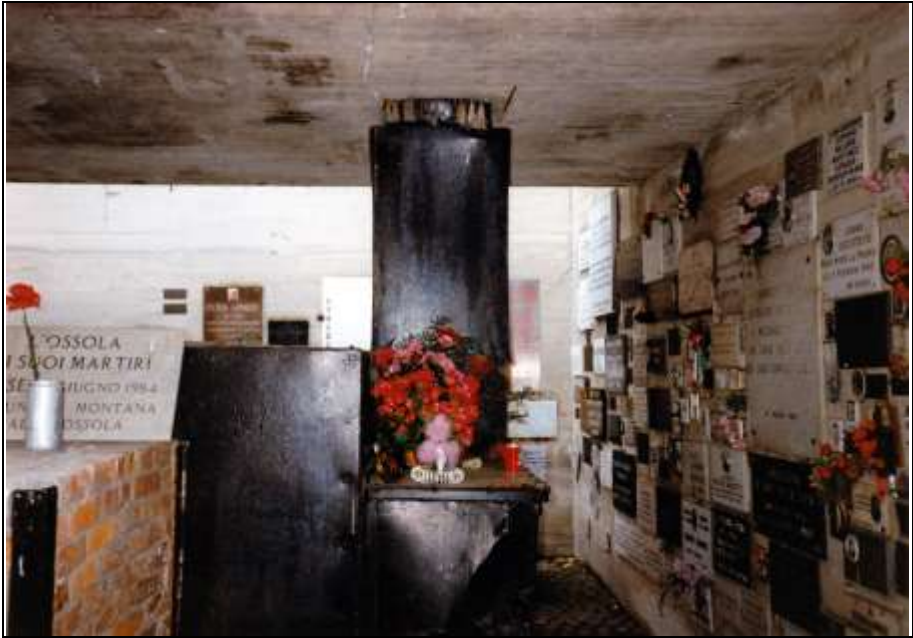
Photograph 32: The rear of the furnace with chimney going through the ceiling (right-hand side).
