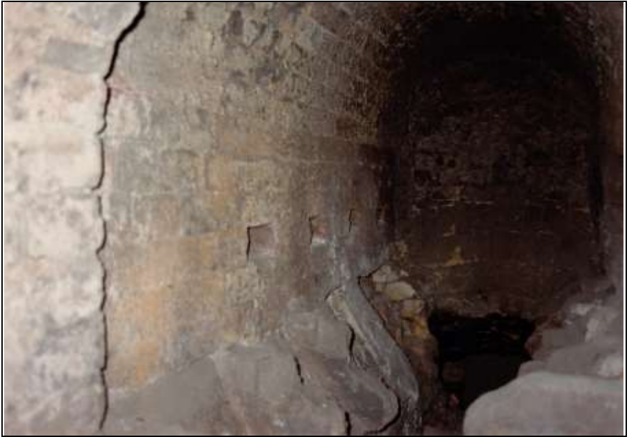
Photograph 141: as above, left-hand muffle wall sloping into the ash chamber with bottom rear opening into the gasifier.
