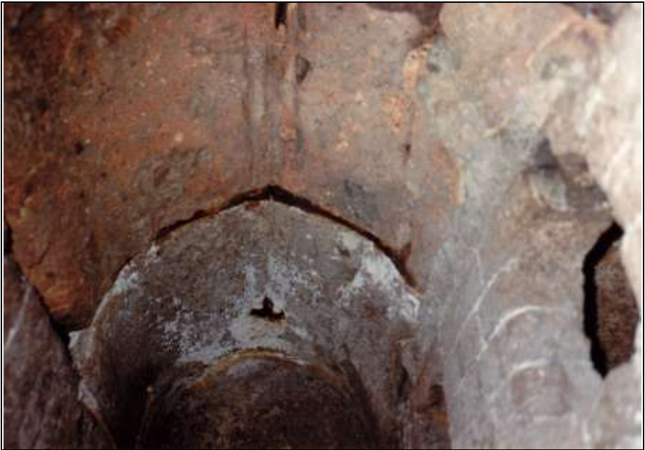
Photograph 19: Left-hand muffle: Vaulted muffle ceiling with the outlet of one of the pipes connected to a blower.
