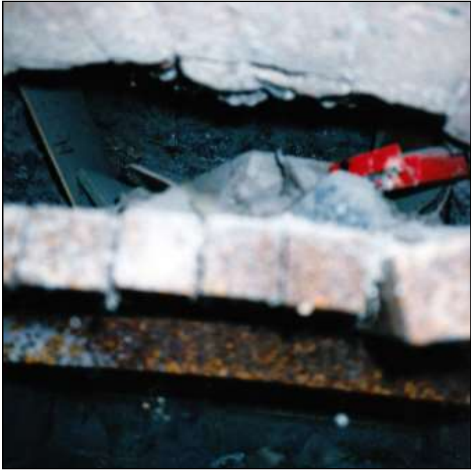
Photograph 82: Grate of the left-hand gasifier (viewed from the rear).
