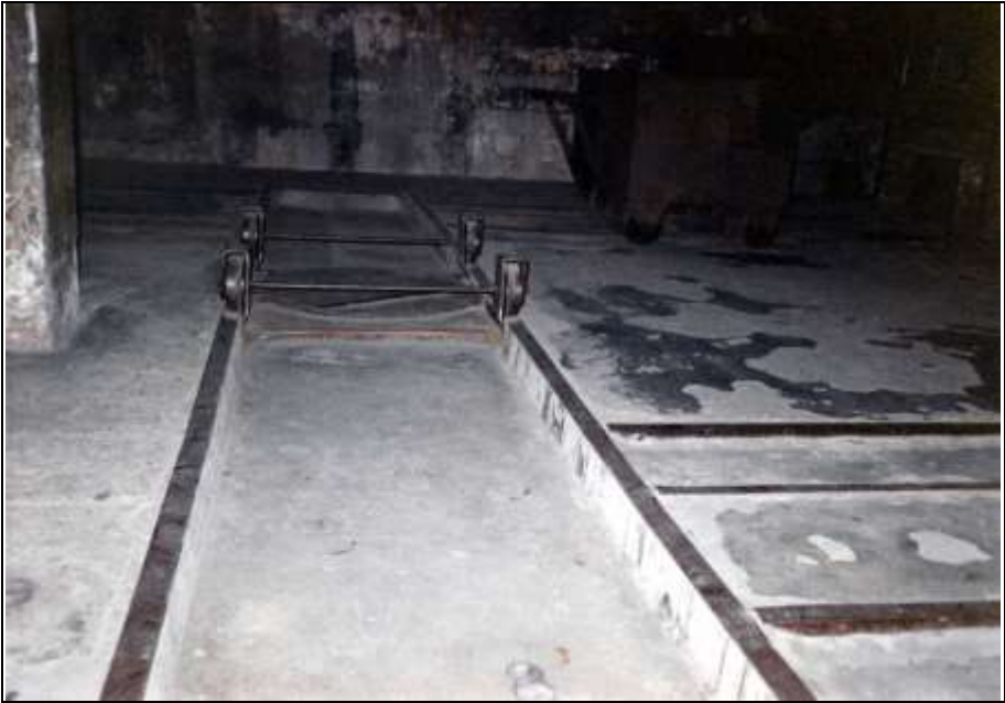
Photograph 105: Transverse rails and rotating platform (turntable).
