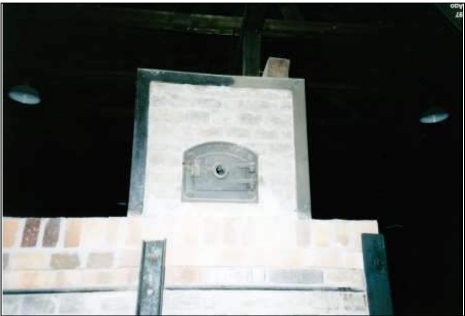
Photograph 310: as above, smoke duct with inspection door.
