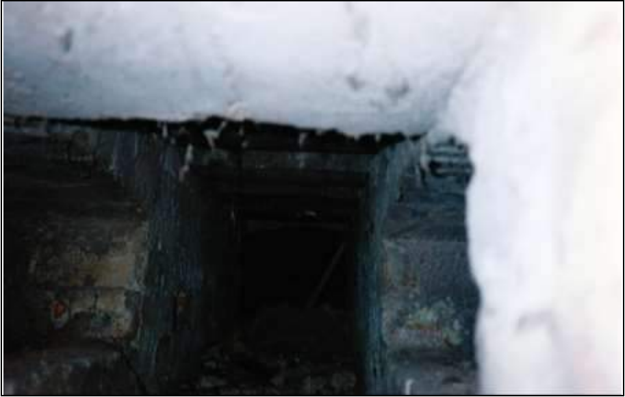
Photograph 72: Ash chamber of the left-hand muffle; at the top the bars of the muffle grate. On the left in the rear part of the wall are two small square openings of a combustion-air intake connected to a channel which opens on the left side of the furnace (see Photos 73f.). In front of those openings is the large opening of the flue-gas outlet; to the right the large opening connects to the ash receptacle of the right-hand muffle.
